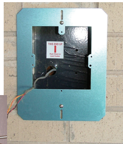
Figure 6 - DMCFR installation
