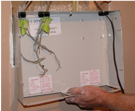
Figure 2 - dmc1H or dmc1HC wall housing placement
